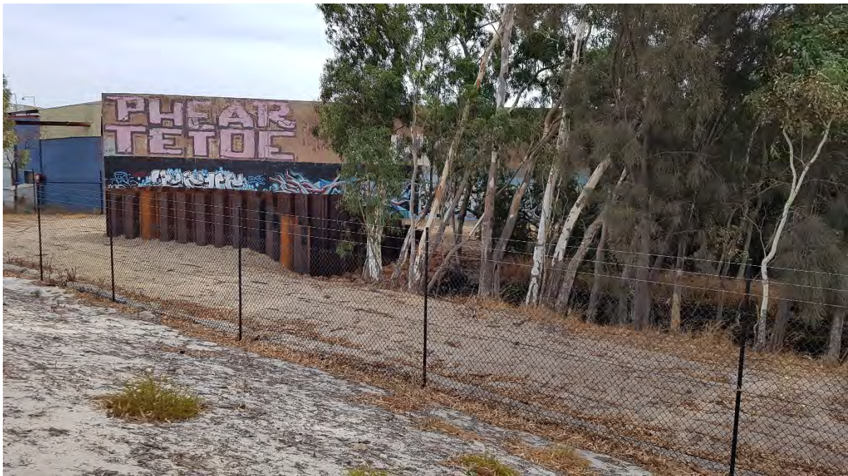
Photo 3. View west showing steep embankment to Tonkin Road (and possible uncontrolled fill). Photograph taken from eastern road verge, in the southern portion of the site.
