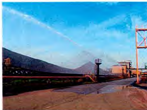
Plate 4.3 Water Sprays on Ore Stockpile at Kakogawa
