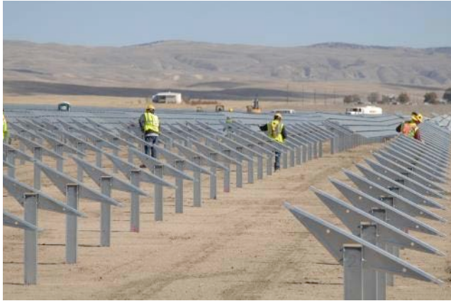
Plate 2.11: Typical solar panel rack installation.
