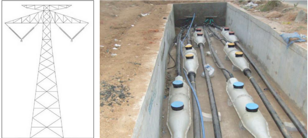
Figure 2.24: Example overhead HVDC pylon and cable burial jointing bay.
