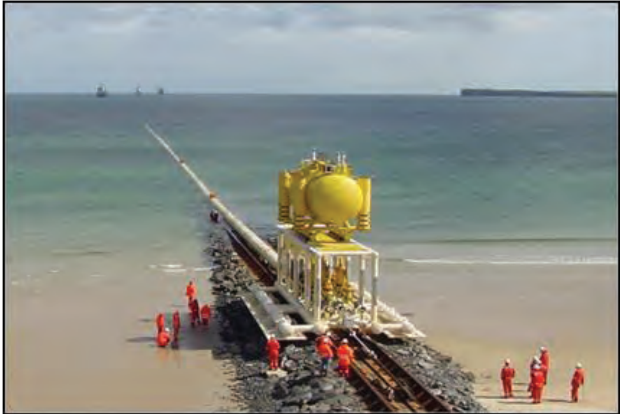
Figure 1.2 Indicative image of launchway structure from Wick with pipeline being launched
