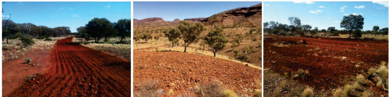
Figure 11. Examples of light disturbance rehabilitation. Left: Track scarification (ripped). Centre: Contour blending. Right: Topsoil and vegetation return on drill pad.
