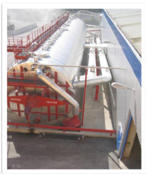
Figure 7 Example of a Horizontal Dry System Digester
