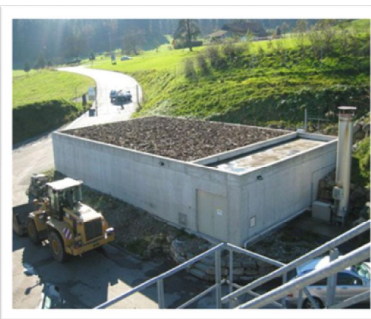
Figure 9 Example of a Biofilter
