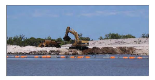
**Plate 2**. Removal of coffee-rock confining layer following prior removal and stock piling of top-soil (1 m) and over-burden.
