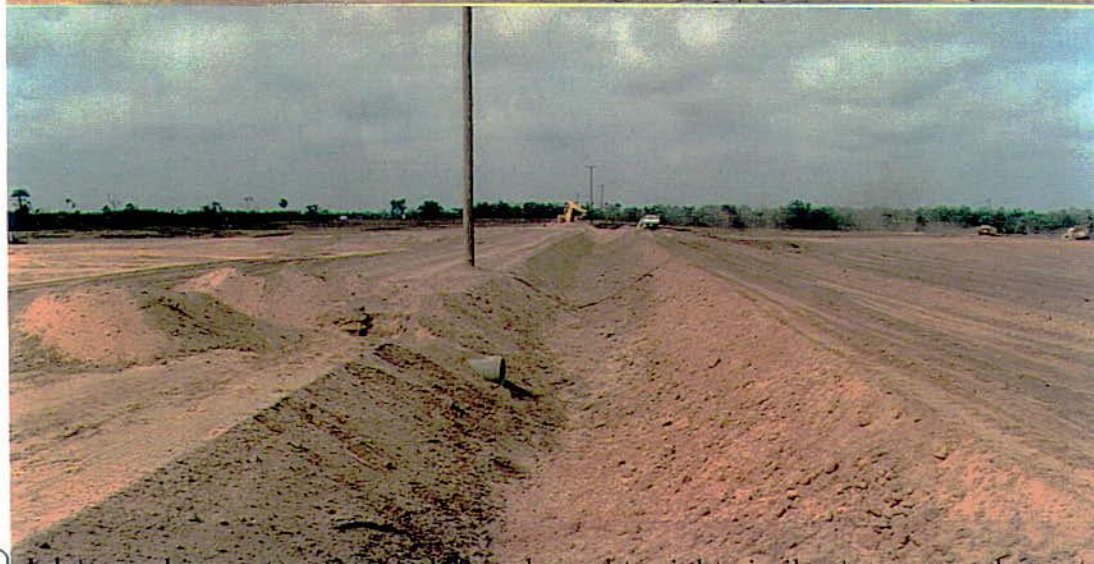
Figure 7 Inlet canal in centre, road to left and pond to right similar to proposed construction.
