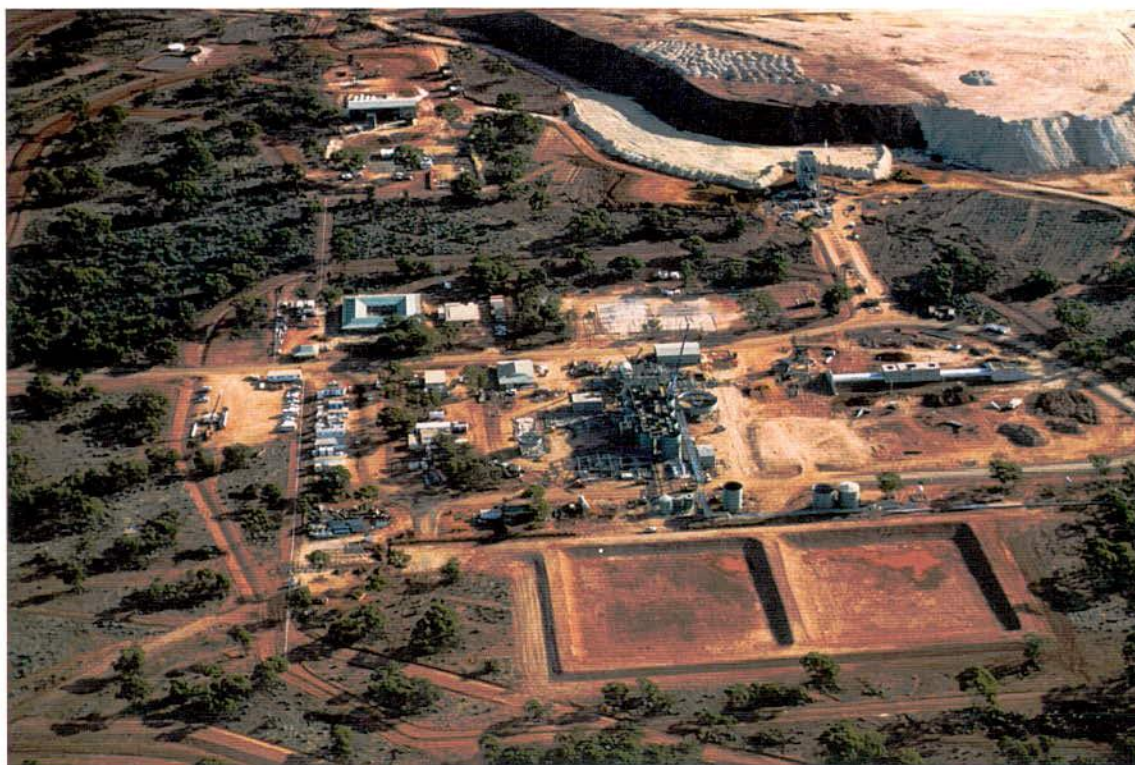
The Kanowna Belle Project with construction of the plant in progress. The concentrates storage dam and the process water dam are in the foreground.
