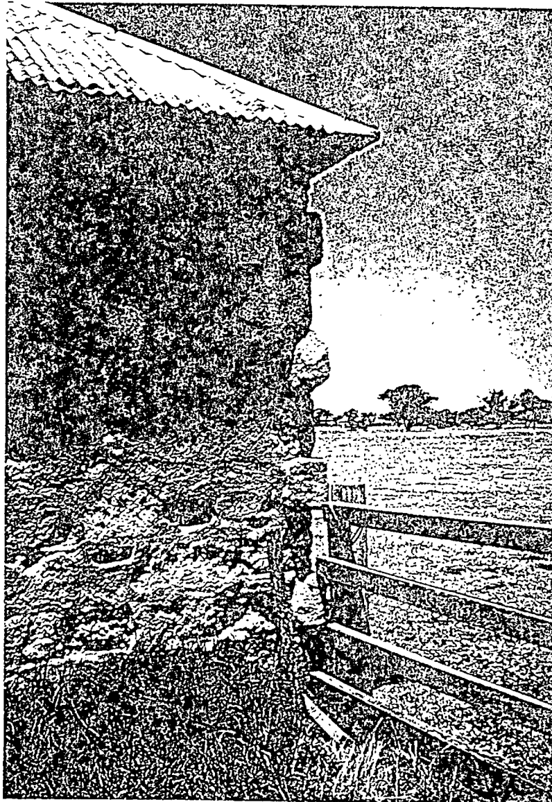
PHOTOGRAPH N° 10 Northern end of the Men's Sleeping Quarters, showing projecting corner stones for future extensions.
