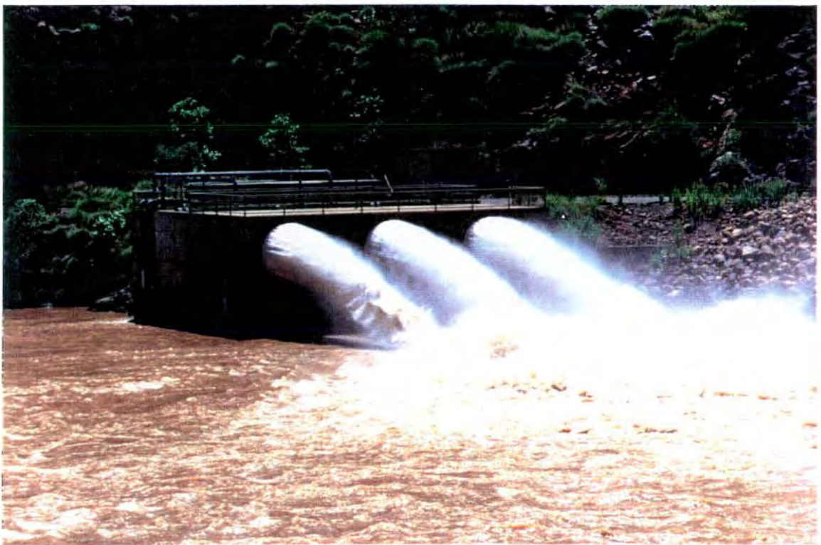
The irrigation valve block located at the toe of the Ord River Dam. Discharge can be regulated from one or all valves, and at the time of the photograph all three valves were open 5%.
