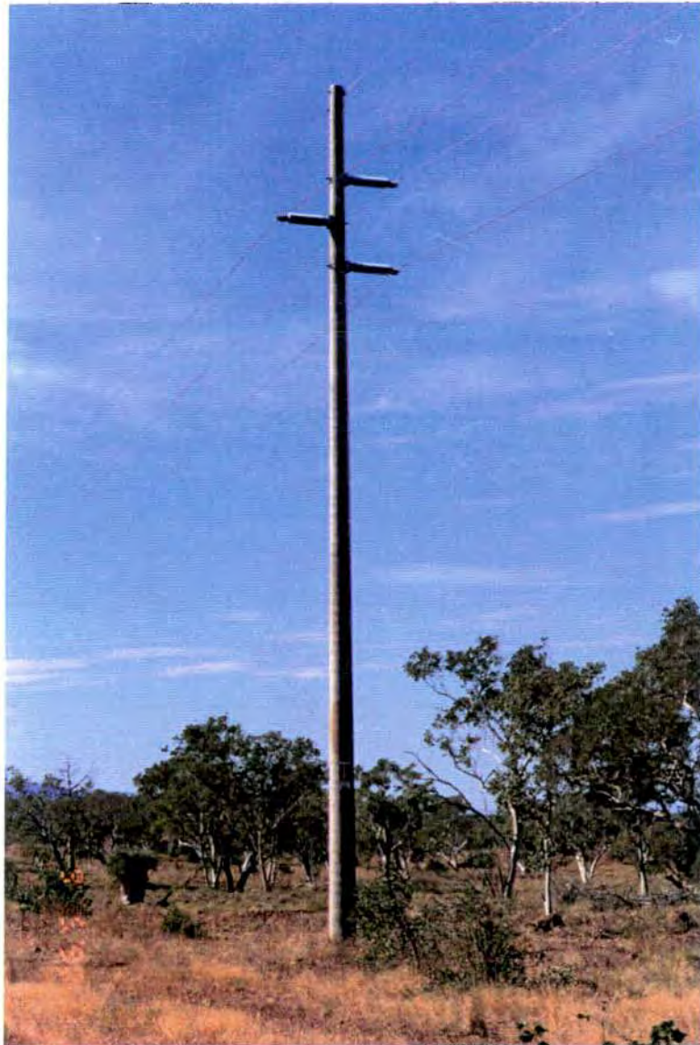
A typical power line pole and insulator arrangement, similar to that proposed for the transmission line to the Argyle diamond mine.
