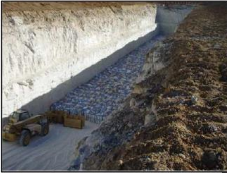
Figure 3: Example of placing intractable waste into the excavated clay slot at the Mt Walton IWDF (Dept. of Finance, 2014).
