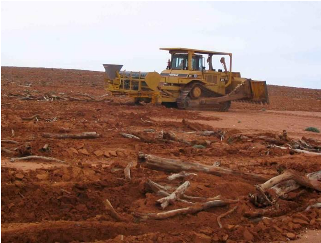
Figure 17: Example of using tree debris on a freshly reinstated sandy topsoil on a waste dump to minimise wind erosion in Western Australia.
