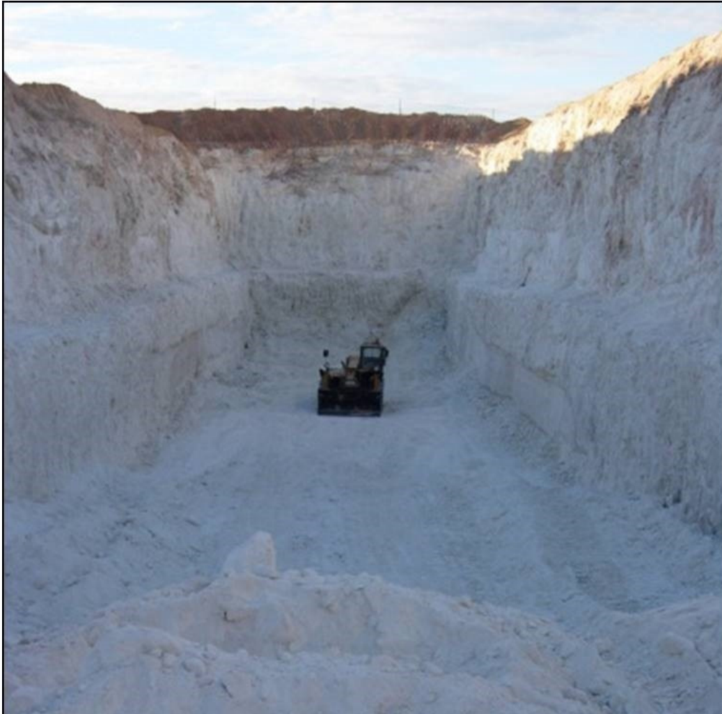
Figure 7 Pit at Mt Walton East Waste Disposal Facility cut down through the mottled zone into the kaolinite zone (Dept of Finance, 2013)
