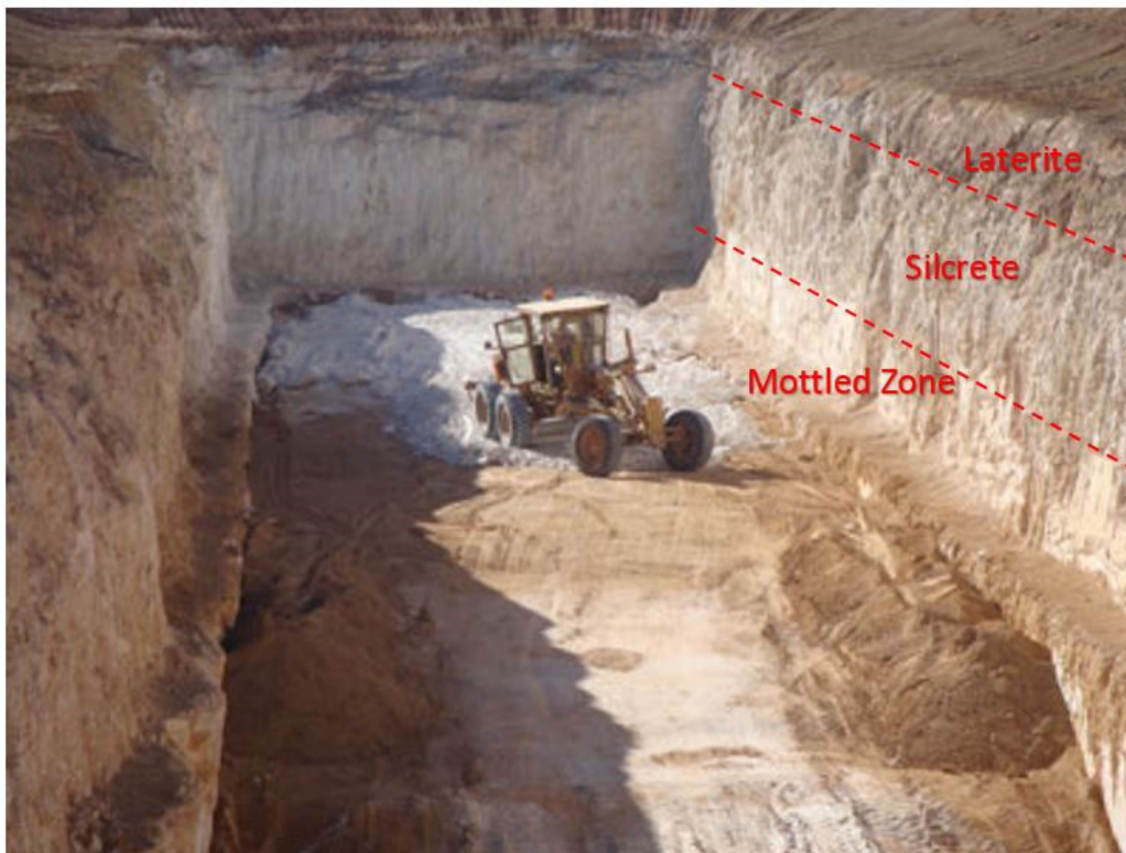
Figure 6 Pit at Mt Walton East Waste Disposal Facility cut down through lateritic and silcrete layers into the mottled zone (from Dept of Finance, 2016)
