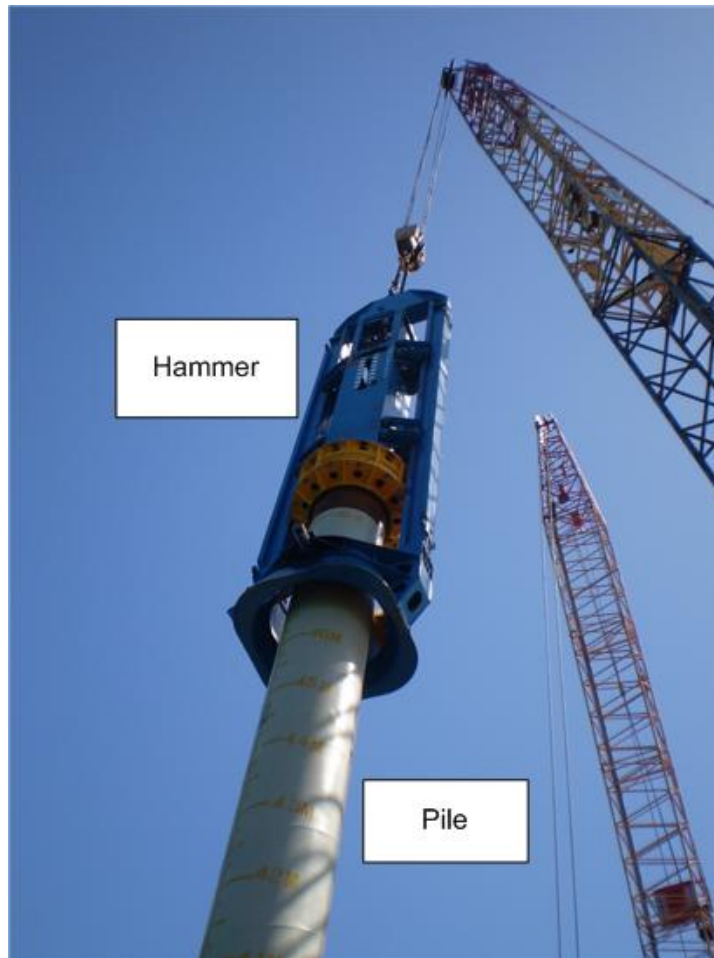
Figure 1-2 A photograph of a pile with a hammer on top (photo taken at Cape Lambert for a 1200mm steel pile).
