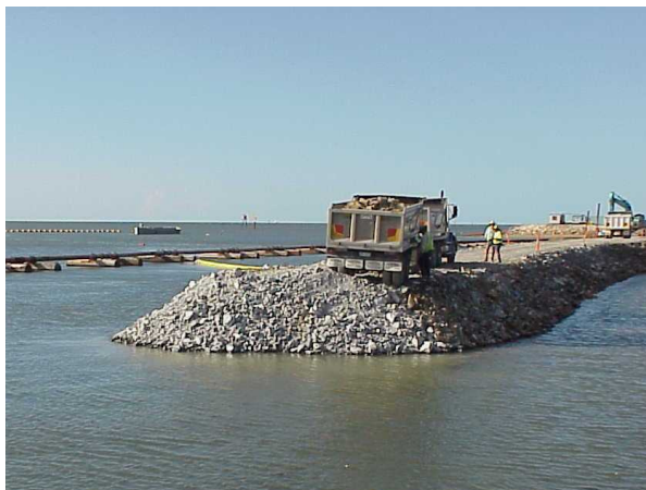
Figure 14 - Aerial and ground level views of bund wall development similar to proposed method and material. Note that in these photographs, the core of the wall has been placed, with outer armour rock layers to be installed.
